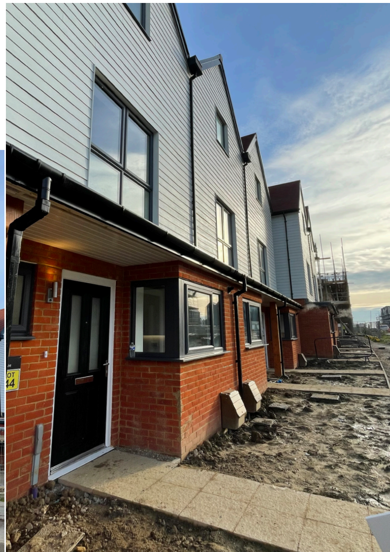
Images depicting homes and construction within the Chilmington development.
